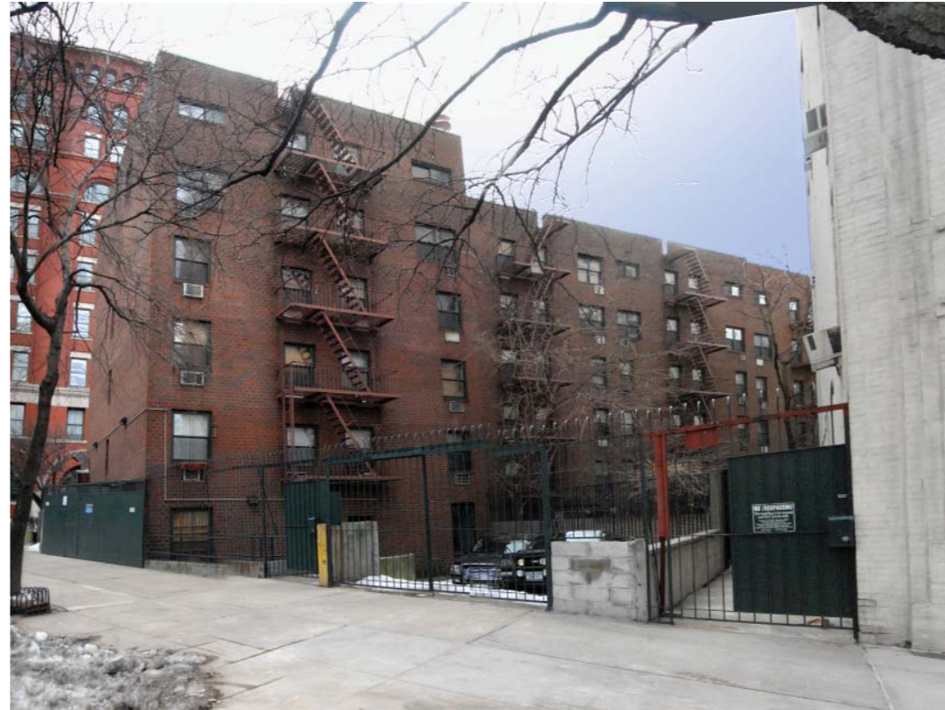
view of existing courtyard
