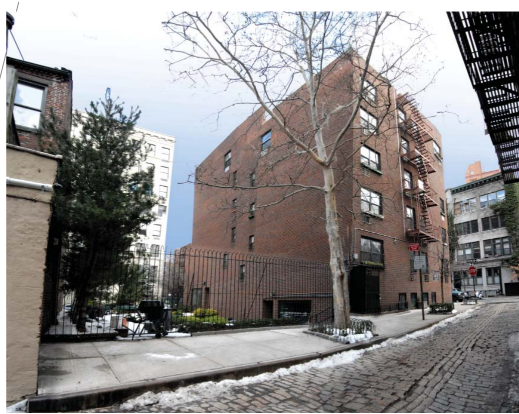
view of existing courtyard
