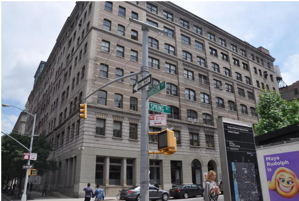
304 Hudson Street, one of several buildings that make up the parcel purchased by Disney. | PropertyShark
