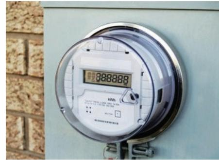
“Smart” meter with digital readout
