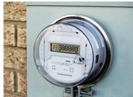
“Smart” meter with digital readout
