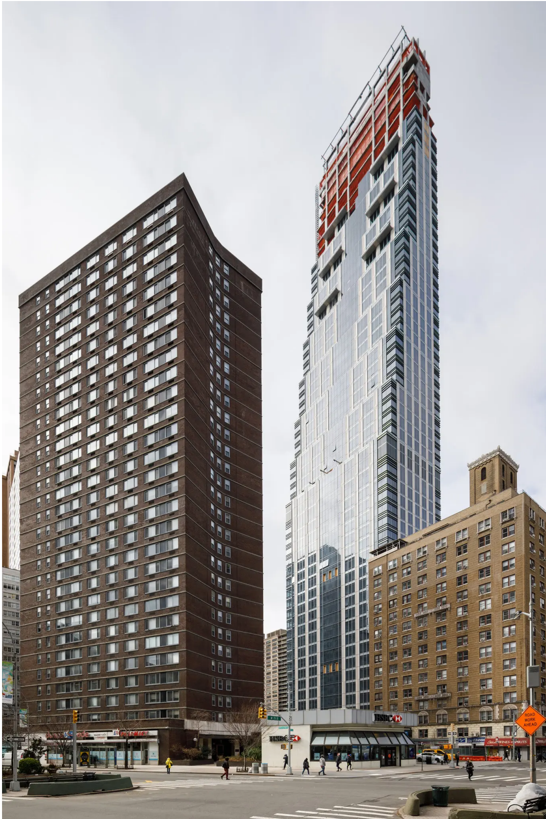
The nearly finished tower at 200 Amsterdam, on the Upper West Side, could face consequences — perhaps even the removal of some high floors — for using what critics call a “gerrymandered” zoning lot to achieve its height and bulk. Stefano Ukmar for The New York Times
