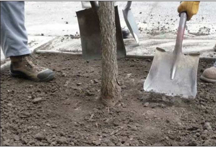
This tree was established at the proper grade after finding root flare.
