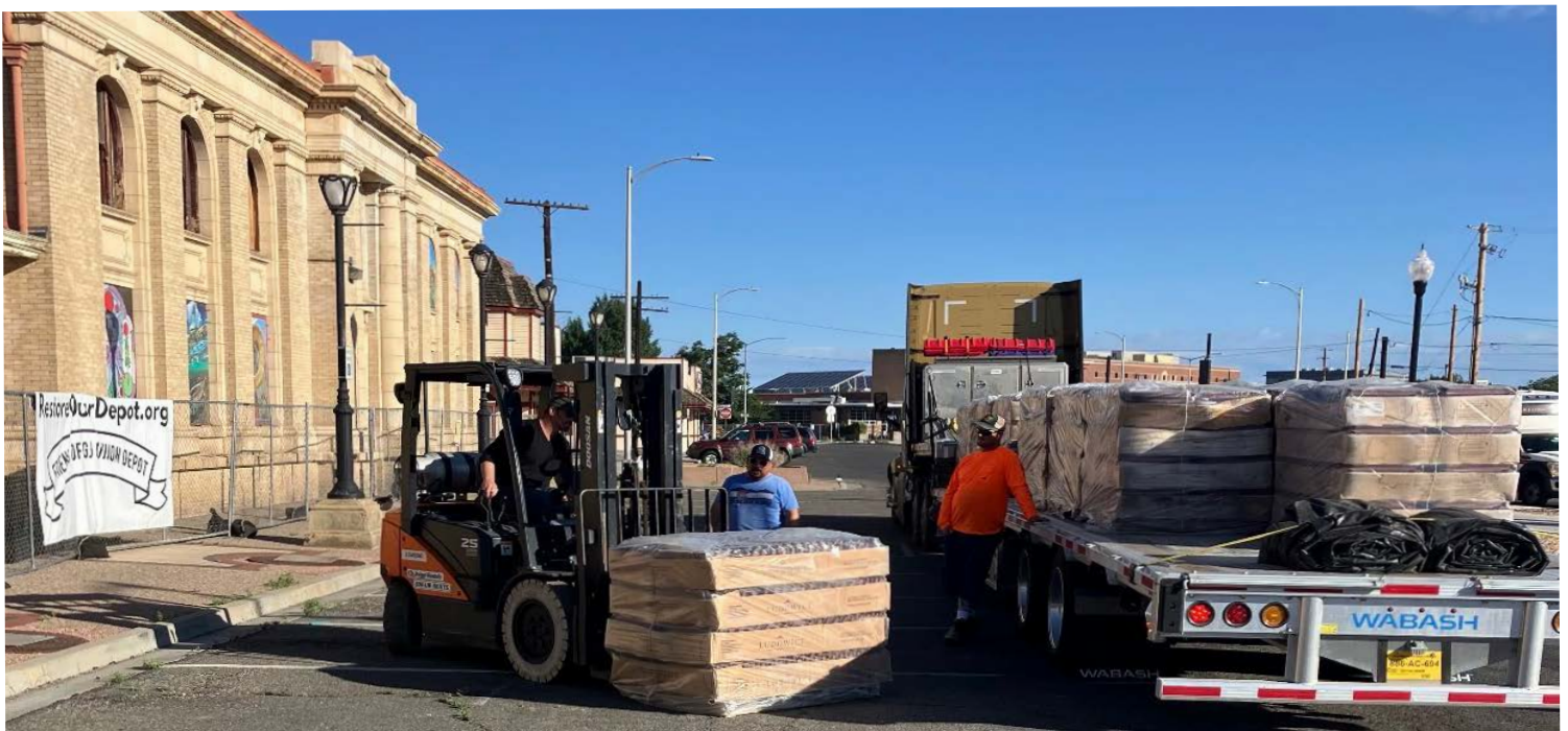
New roof tiles are unloaded at the Grand Junction Union Depot.
