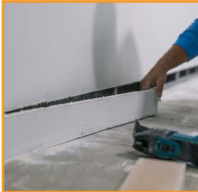
Prep Site Remove excess & mark studs
