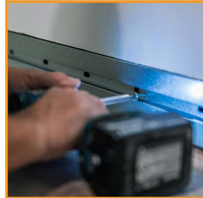
Secure StepStuds™ Screw studs in place
