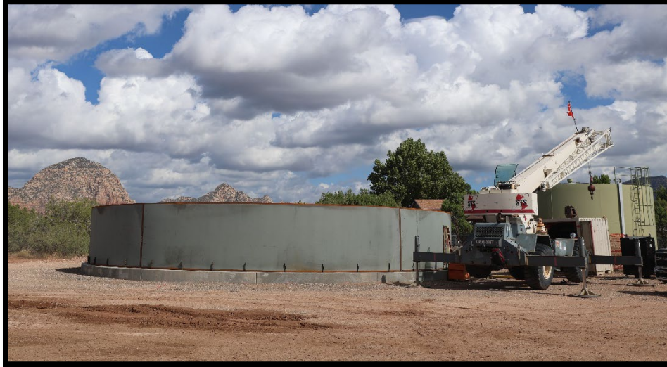
FSWS Tank Erection
