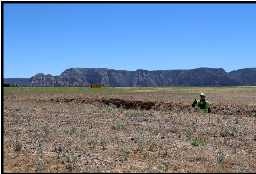
Infield Ditch Erosion
