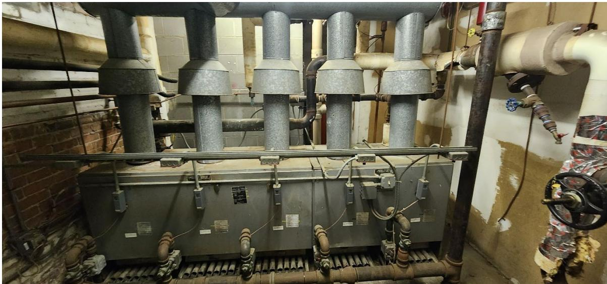
There are two 250,000 btu/hr input gas fired 98 gallon water heaters located in a mechanical room on the fourth floor.
