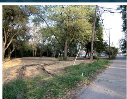
Trailer Park Demolished
