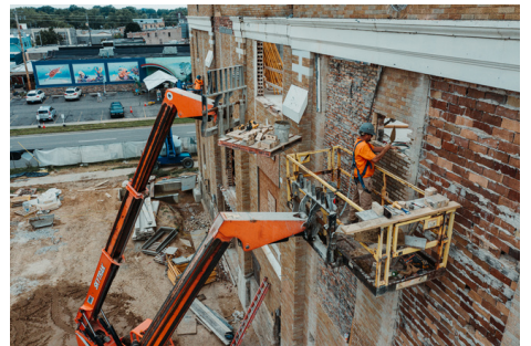
Temple Lofts Under Construction
