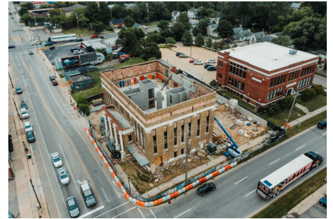
Temple Lofts Under Construction
