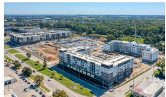
Red Cedar Under Construction
