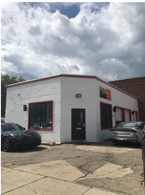
629 N. Butler After Photo (New paint, signage, lighting, and update garage doors.)
