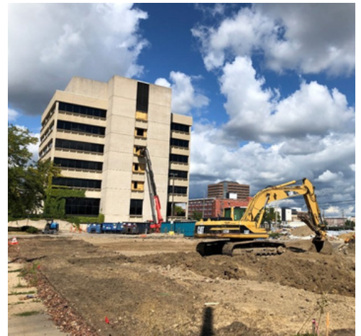
City View While Under Construction
