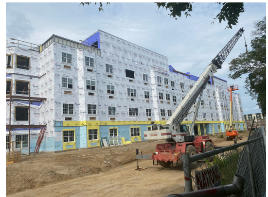
Red Cedar Under Construction
