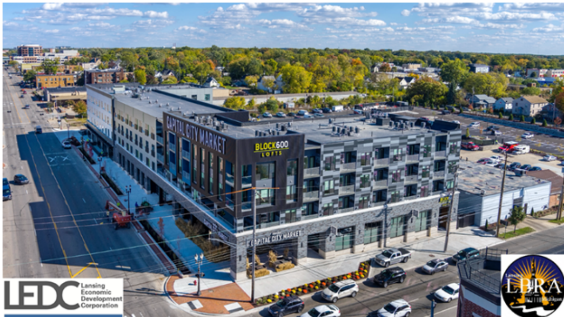
The Award-Winning BLOCK600 Project in Lansing
