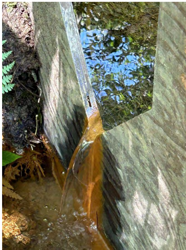
Vee Notch Weir for MC2 Showing Low Flow Conditions
