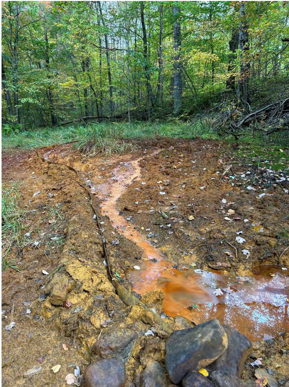
MC3 Mine Discharge Showing the Channel Built to Consolidate the Flow.
