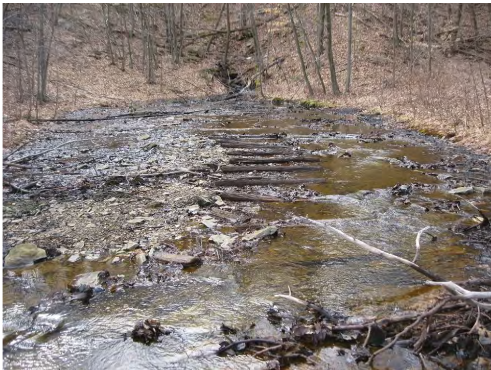
Water Flowing From a Collapsed Mine Entrance in the Bear Run Watershed.
