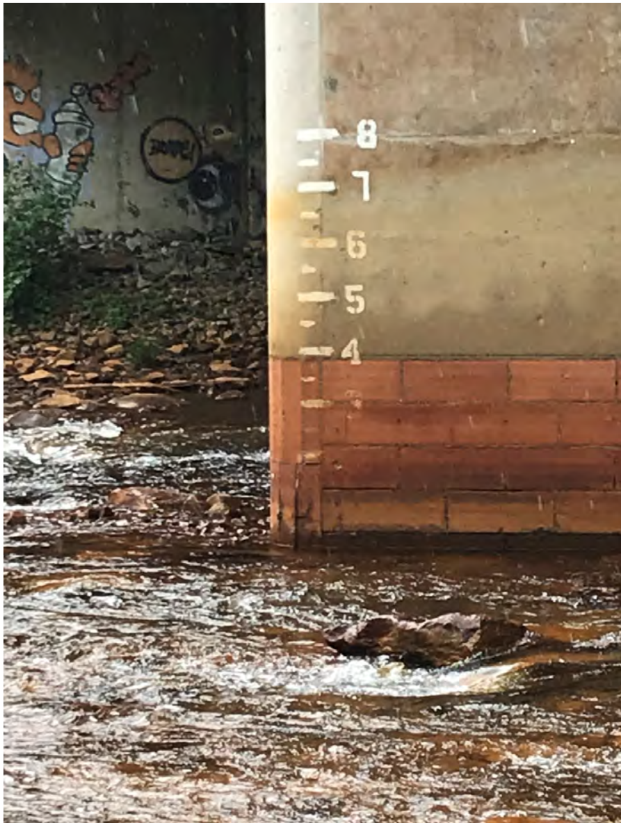
Figure 14. Moshannon Creek low flow condition on July 11, 2020 at Hwy 53 Bridge.
