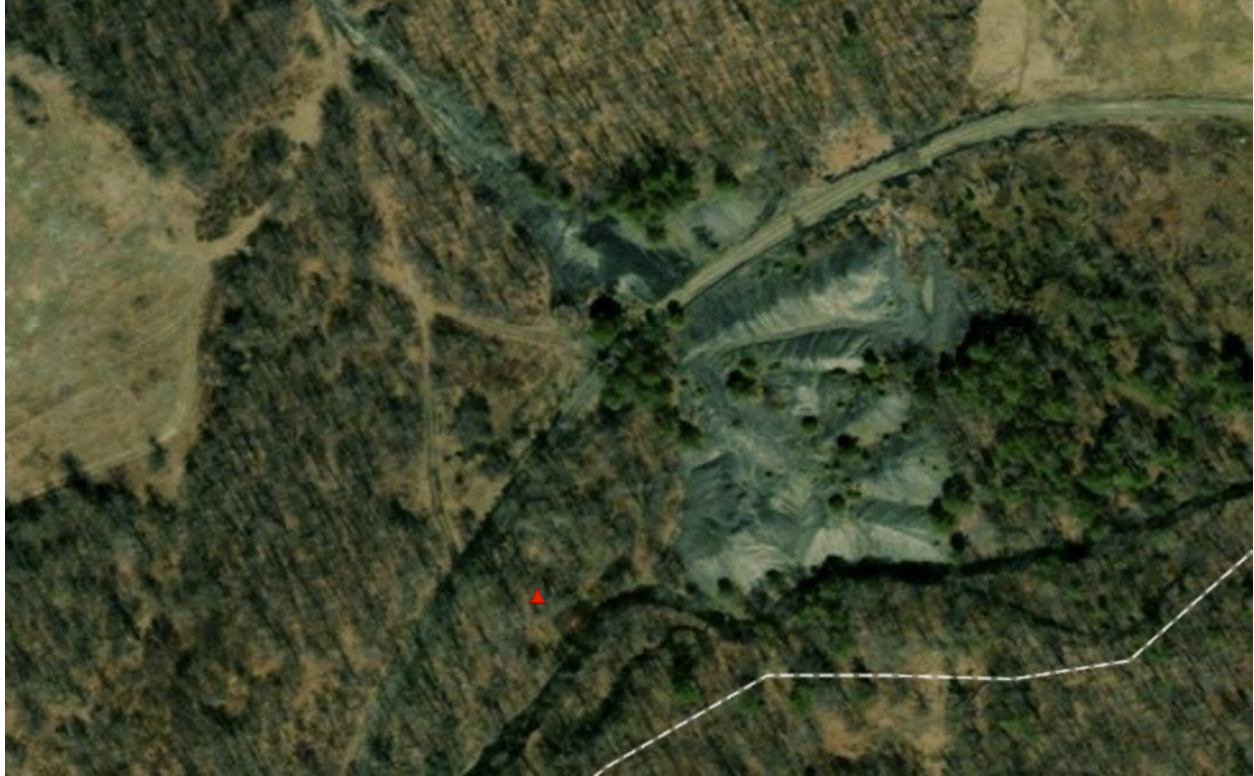
MC3 Discharge and Coal Refuse Pile. From the SRBC Website.
