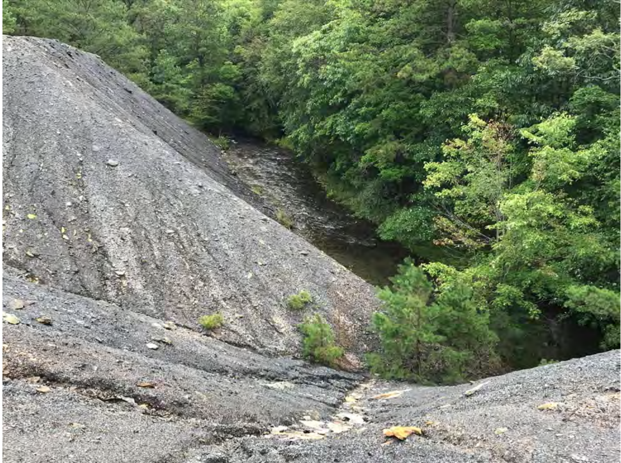
Coal Refuse Pile Serving as West Bank of Moshannon Creek near Wilson Run. 8/31/2021.
