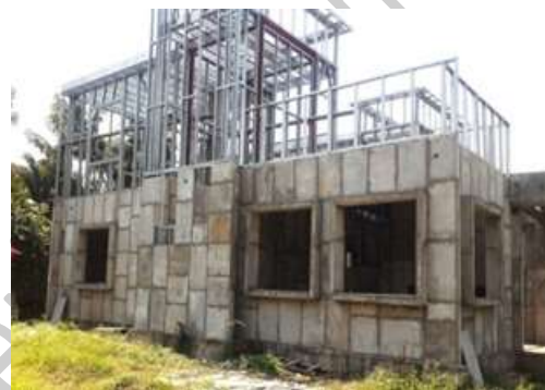
Fig. 3. Photographic view of partially completed composite building.
