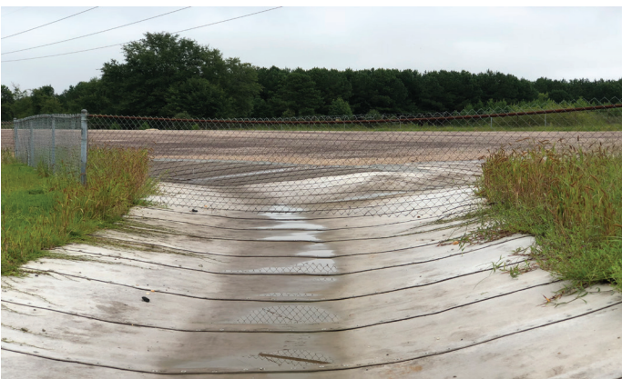
Newly covered swale using Concrete Cloth GCCM
