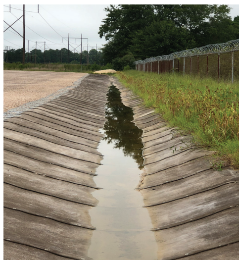
Newly covered swale using Concrete Cloth GCCM
