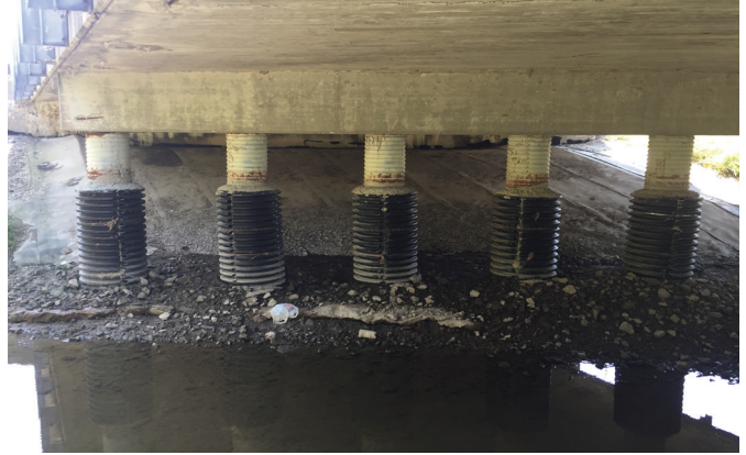
Completed installation three years later, view from opposite bank.
