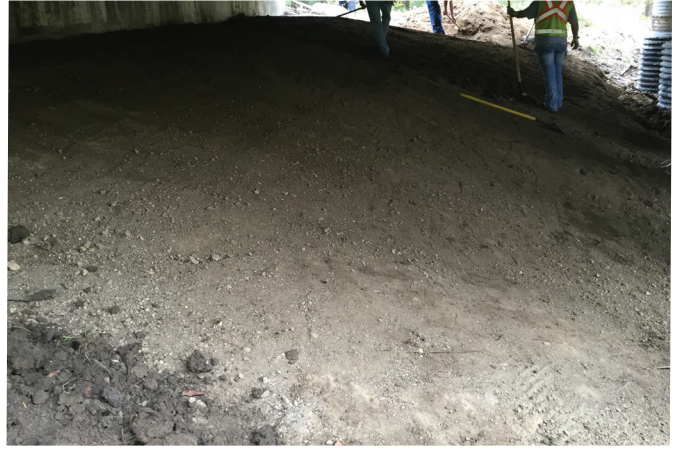
Surface restoration prior to Concrete Cloth GCCM installation.
