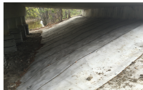
Completed Concrete Cloth GCCM installation.
