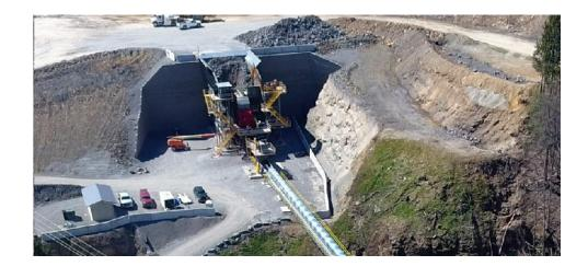
A new primary crushing station has been constructed at Allegheny Mineral Corp.'s Mine 24 in Slippery Rock, Pennsylvania. Construction of the station involved installation of a Keystone Compac III segmental retaining wall system to create the concrete dump pad at the top of the retaining wall. From the pad, 200-ton offhighway trucks capable of hauling 116-165 cubic yards of rock dump their loads into the hopper of the crushing tower situated at the base of the 47-foot-high wall.
