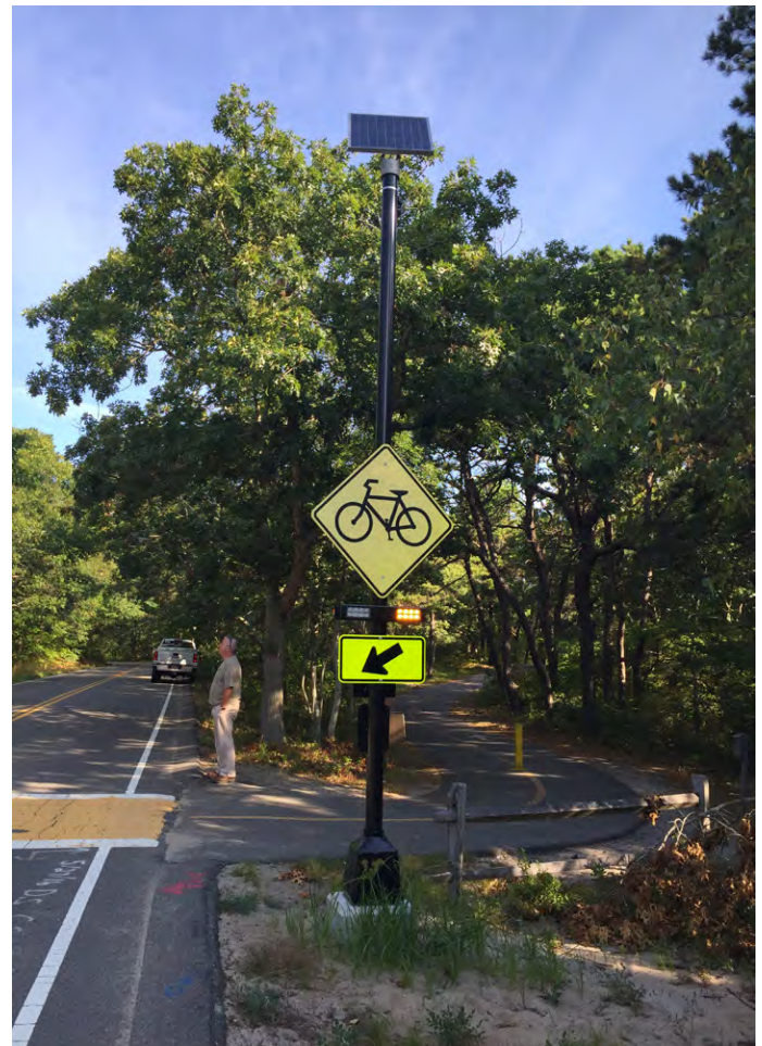
Figure 3-18: A flashing beacon signal at a trail crossing in the Cape Cod National Seashore in Massachusetts. (Source: NPS)
