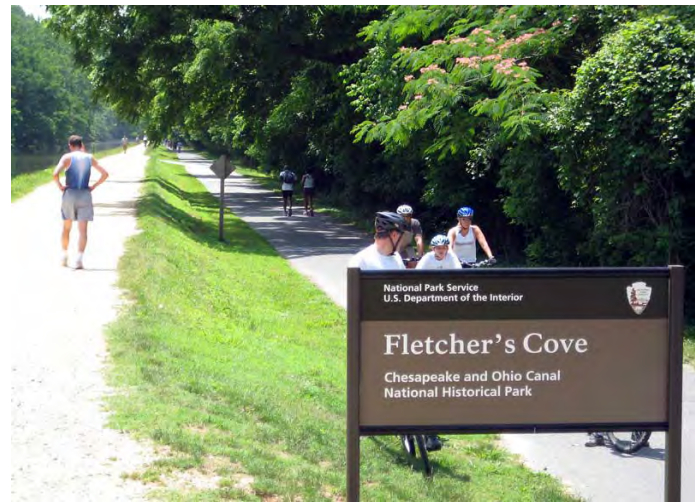
Figure 3-14: A multiuse trail at Chesapeake and Ohio Canal National Historical Park in Washington, D.C. includes a gravel path and a parallel paved path to provide options for pedestrians, bicyclists, runners, and others using the trail. (Source: National Trails Training Partnership) 20
