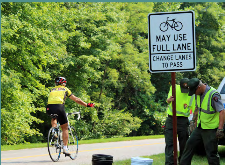
Figure 4-9: NPS employees installing bicycle signage at Natchez Trace Parkway. (Source: NPS)
