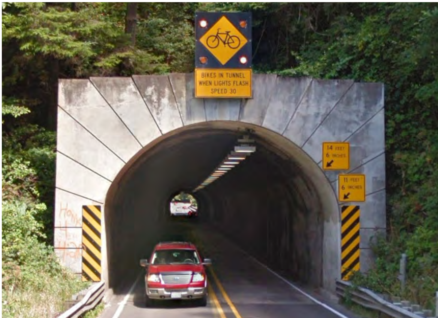
Figure 4-5: Bicyclist-activated dynamic warning signals indicate to vehicles that bicyclists are present on the road. (Source: Google Streetview)
