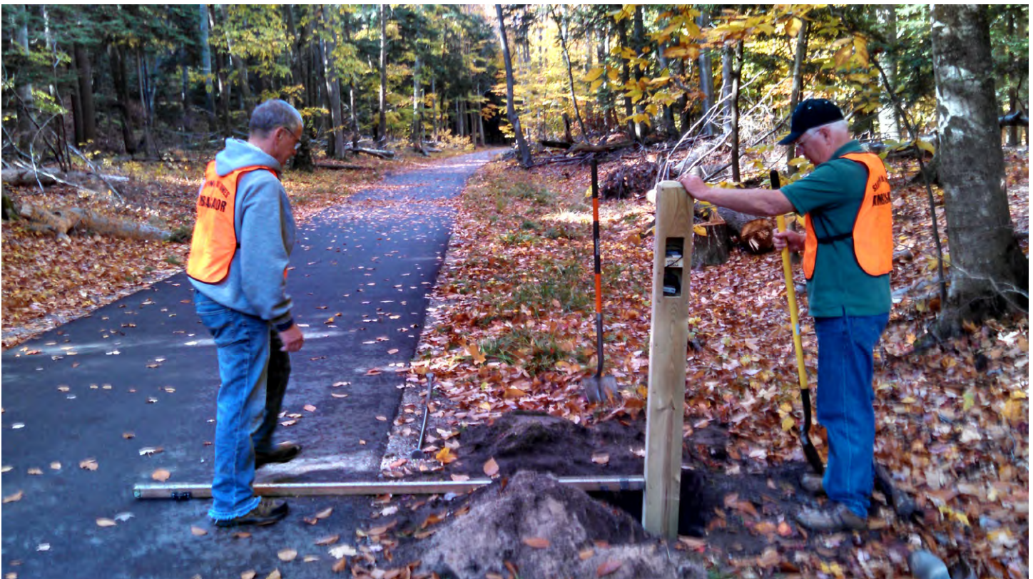
Figure 10-2: Installation of a pedestrian counter at Sleeping Bear Dunes National Lakeshore. (Source: NPS)
