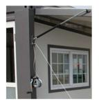
After ensuring that the cable is securely hooked and ready, release the locks on the floor panel. Give a gentle push from inside the unit to set the movement in motion. Lower the floor slowly and steadily using the hand winch.
