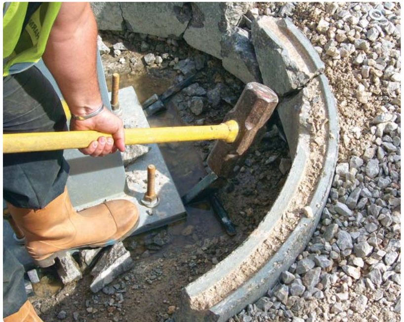
Figure 1: Striking of steel wedges with sledgehammer to force bolts into correct position.
