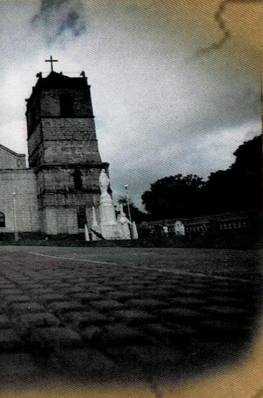
Completion of the Castle Church
