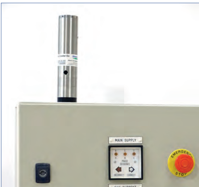
EX Cabinet cooler fitted to an electrical panel.
