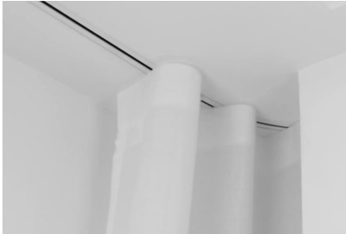
Trackrim® Curved Section finished installation.
