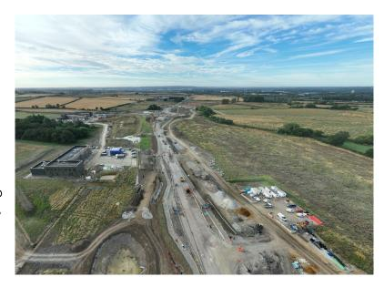
The removal of the temporary bridge south abutment on Newport Road is nearing completion and the new eastern link road network is taking shape. Earthworks are continuing towards the direction of the M1 with drainage works ongoing. Both subways in this area have been waterproofed and the backfilling continues.
