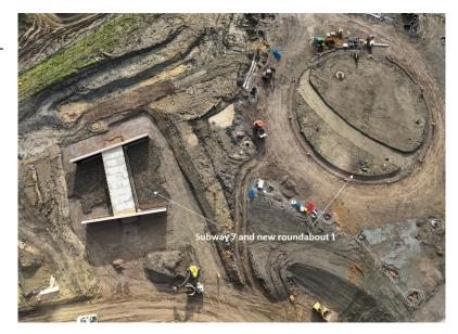
We are making good progress on site. The construction of our third roundabout out of five is underway and the installation of utilities in the new redways is ongoing. The new temporary alignment along Newport Road is progressing well to allow for the switchover of traffic in October.
