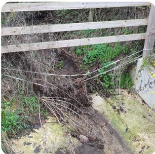
As the name suggests, this area is the lowest point of the land which also has a busy road running through it. Water would collect at this point making it unsafe for drivers especially during winter months when it turns to ice. We worked with the landowner to build an additional trench for water coming off the field and improved the trench to the brook to help carry away the water.
