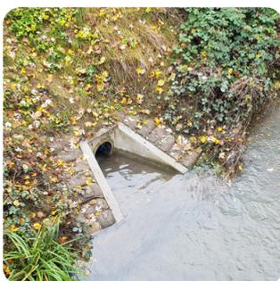
After properties on a nearby road were flooded, the drainage system was checked for problems. We discovered a damaged pipe and tree roots were growing into the pipes too, reducing the capacity to remove water. We removed the tree roots and installed a new pipe and manhole with a headwall. The excess water can also now be discharged into the brook.
