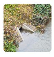
After properties on a nearby road were flooded, the drainage system was checked for problems. We discovered a damaged pipe and tree roots were growing into the pipes too, reducing the capacity to remove water.
