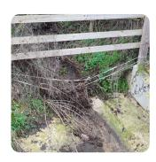
As the name suggests, this area is the lowest point of the land which also has a busy road running through it. Water would collect at this point making it unsafe for drivers especially during winter months when it turns to ice. We worked with the landowner to build an additional trench for water coming off the field and improved the trench to the brook to help carry away the water.
