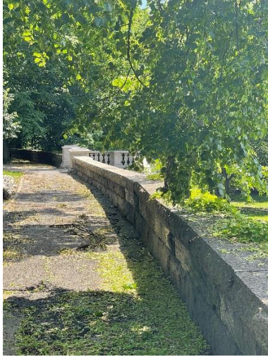
Stairs ahead on right
