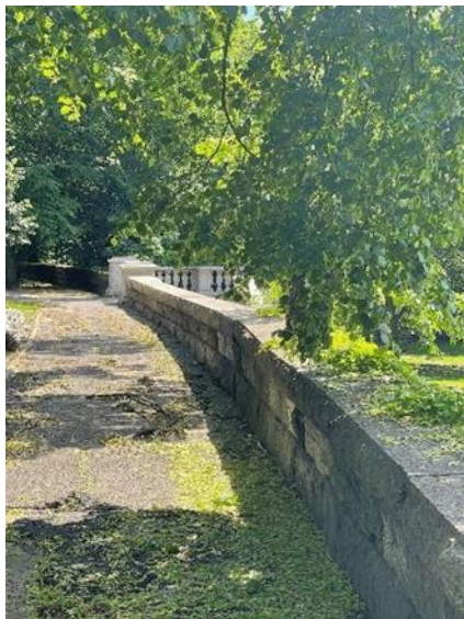
Stairs ahead on right
