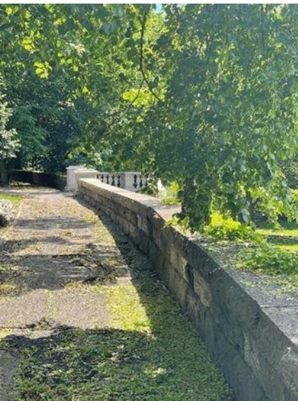
Stairs ahead on right
