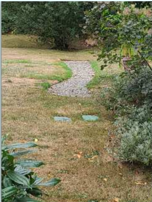
Signs of drainage work at the exterior
