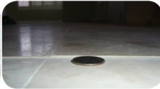
LIPPAGE (UNEVEN TILES)
