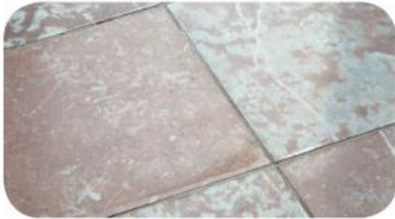
DIRTY, STAINED GROUT LINES
