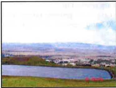
One of the reservoirs that services the Waimea Water Delivery System
