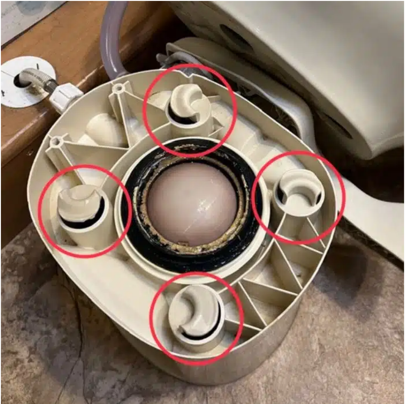
Four holes on the bottom of the RV toilet bowl fit down onto these tabs
