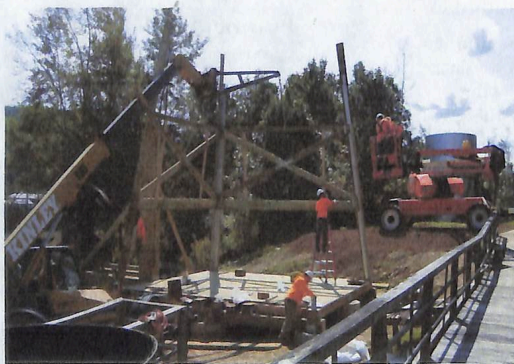
Legs and bracing, going up...
