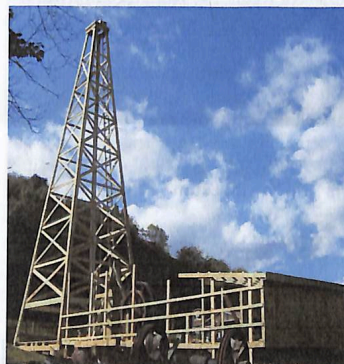
Engine house and belt hall framing
