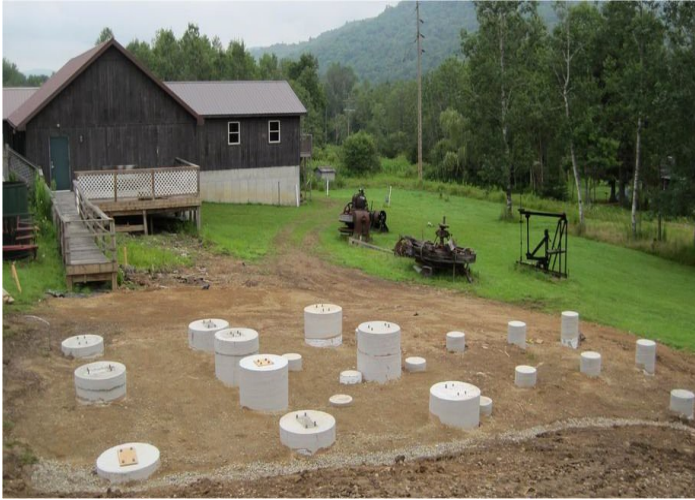
July 2021 - ground cleared and foundations set
