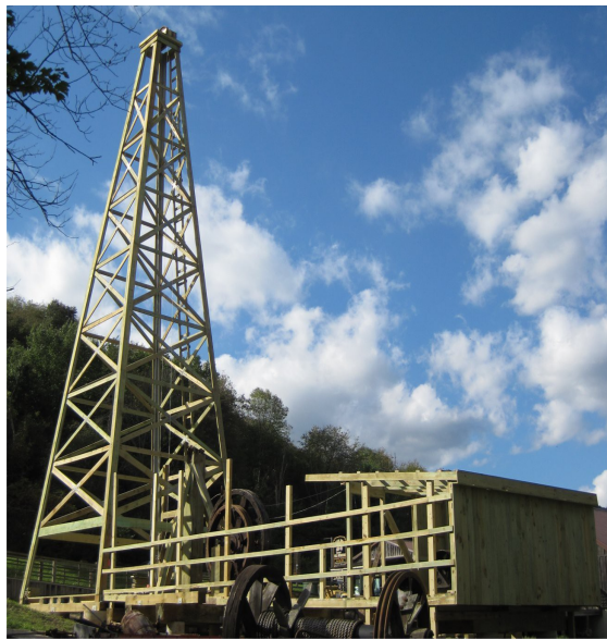
Engine house and belt hall framing
