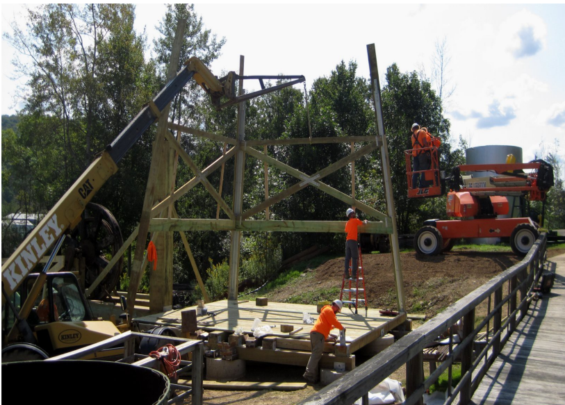
Legs and bracing, going up...
