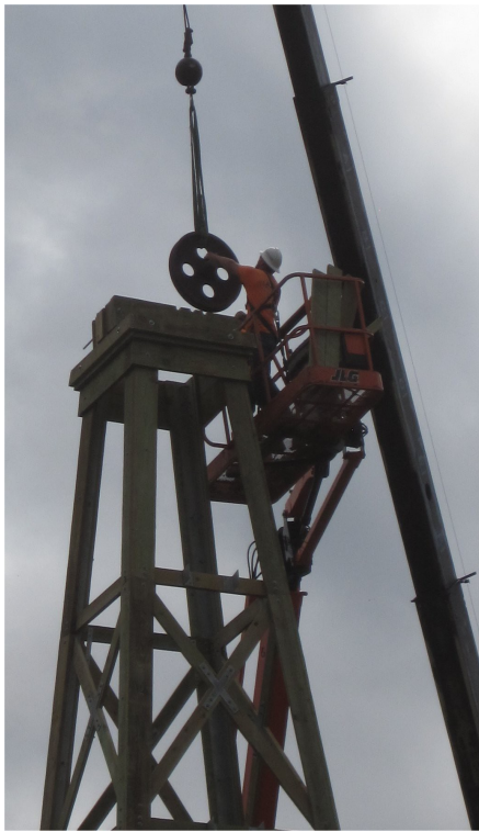
Crown pulley installed
