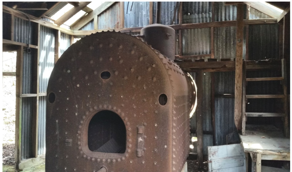
Interior of old boiler house – American Glycerine Plant – Tom Huntoon
