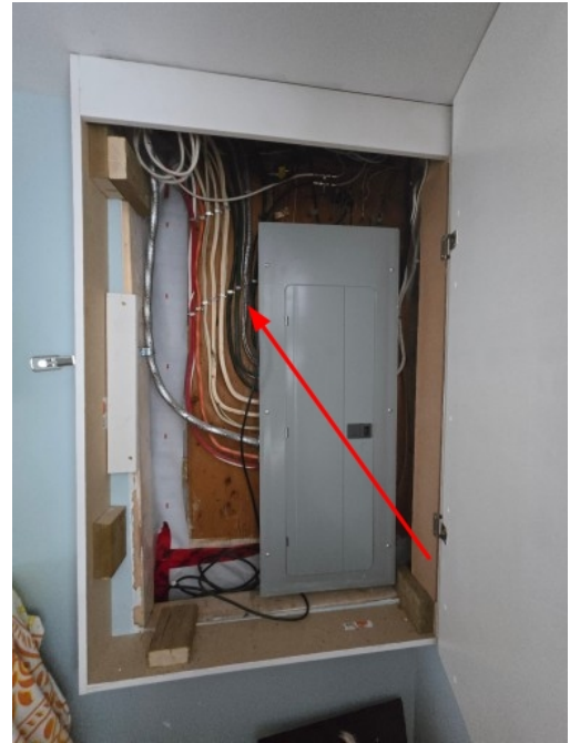
Aluminum branch circuit wiring
