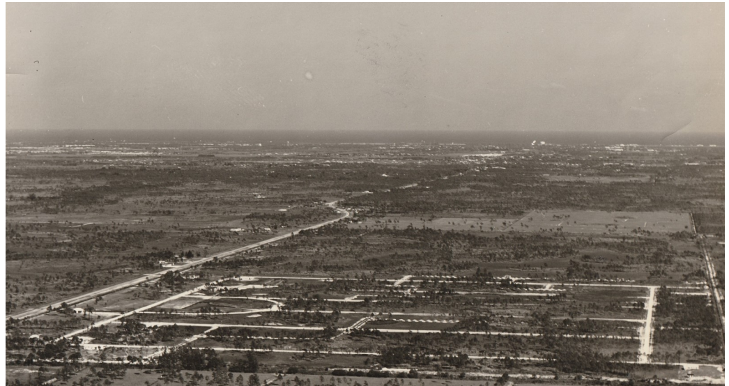
THE WAY WE WERE - A rare aerial view of the north half of Florida Gardens as the roads were being installed in 1954.
