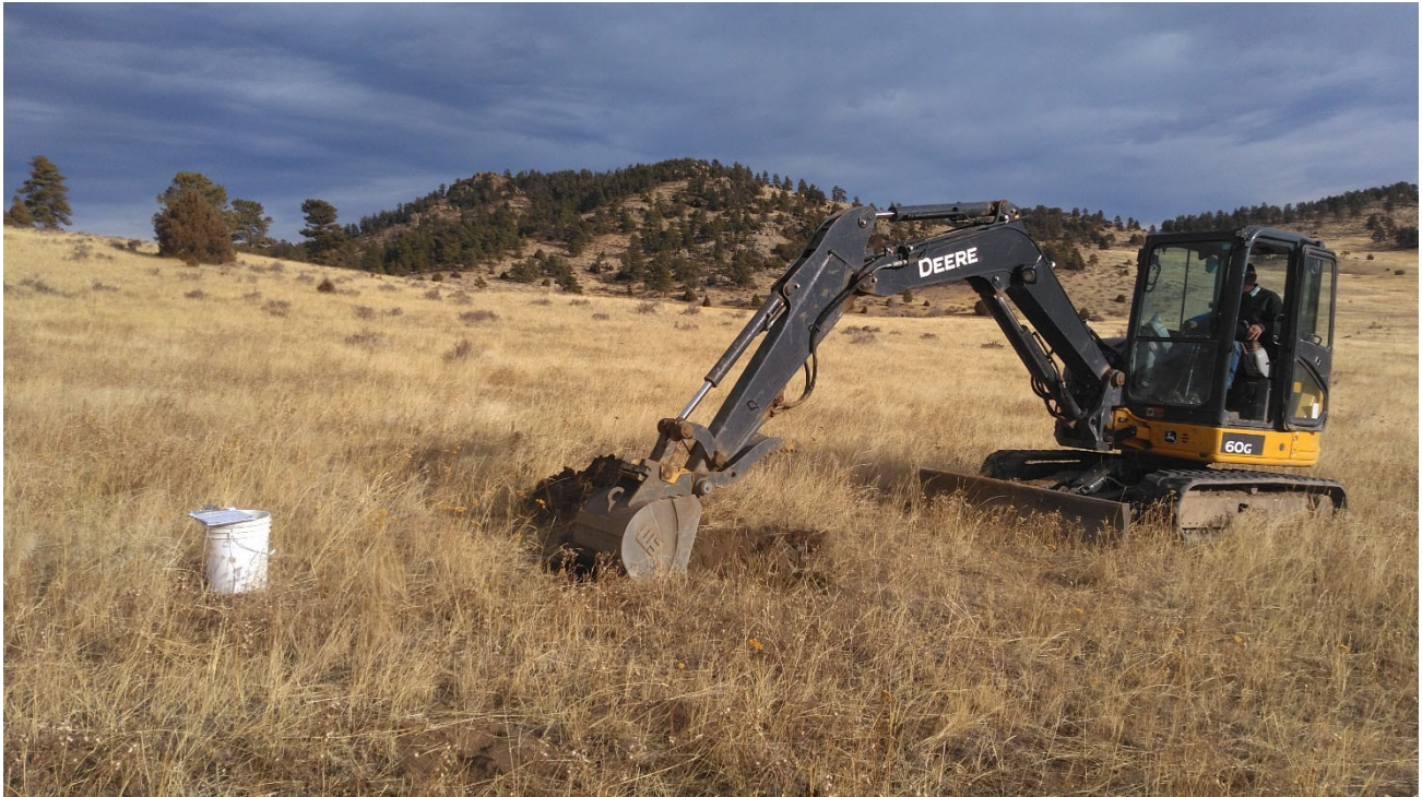
Photo 4. View looking north at Exploratory Pit TP-3.
