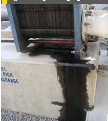
Fig 8: Leaking exchanger gaskets
