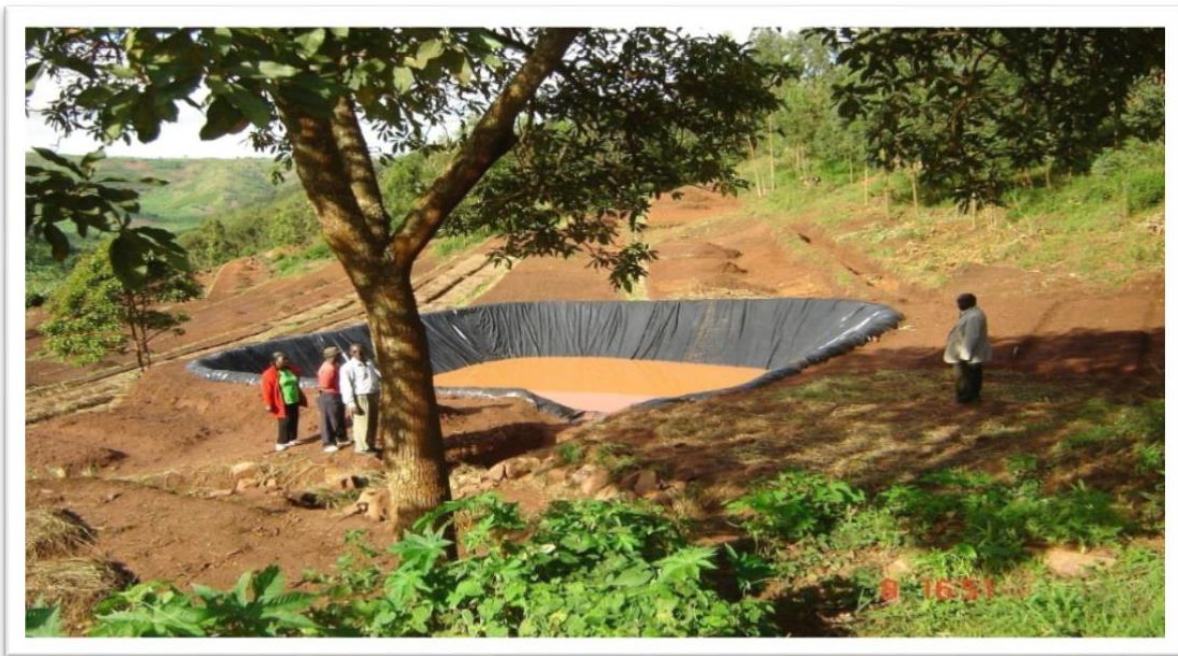
Fig. 1. A pond lined with plastic to reduce seepage and to hold water as a catchment for irrigation and community water use. The photo is to illustrate the pond only- not the removal of trees and vegetation surrounding the pond as was done here in eastern Zambia. The retention of vegetation including shrubs and trees and the least disturbance to the land with the building of a pond area to which your community's excess rain can be channeled is the goal. Soil erosion must be kept to a minimum, all traditional leaders and public policy must be followed so check in advance for permission as needed.
