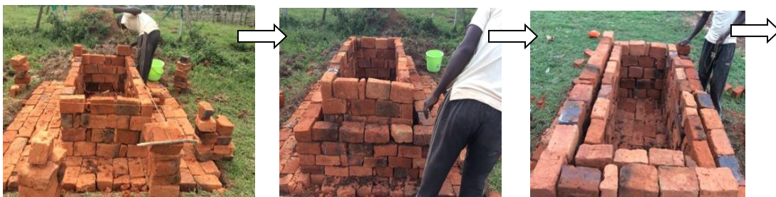
Figure 1: Process of constructing ZECC
