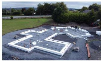
After an initial ground investigation survey on-site, the footprint of the building + 1 m is excavated down to good natural ground. Graded stone fill (typically T3 blinding on T2 permeable on T3 structural) is placed and compacted with services installed as per the project engineer's instructions. The radon membrane is fitted on top of the T3 blinding prior to assembly of the insulated raft, at a later stage the membrane is dressed up on the outside of the insulated raft.
