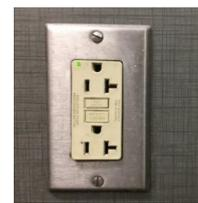
GFCIs are generally installed where electrical circuits may accidentally come into contact with water. They are most often found in kitchens, bath and laundry rooms, or even out-of-doors or in the garage where electric power tools might be used.
