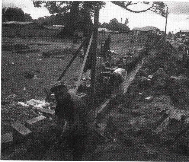
Building the foundations for the fence
