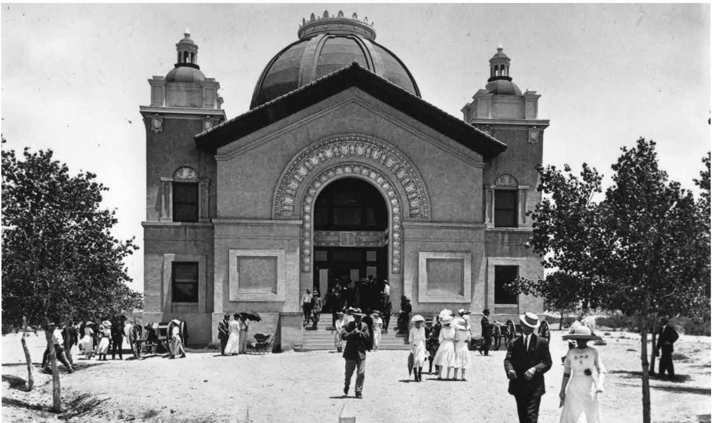
1913 commencement attendees at Trost-designed Hadley Hall on the New Mexico College of Agricultural and Mechanical Arts (now NMSU) campus, completed in 1908 and demolished in 1958.
