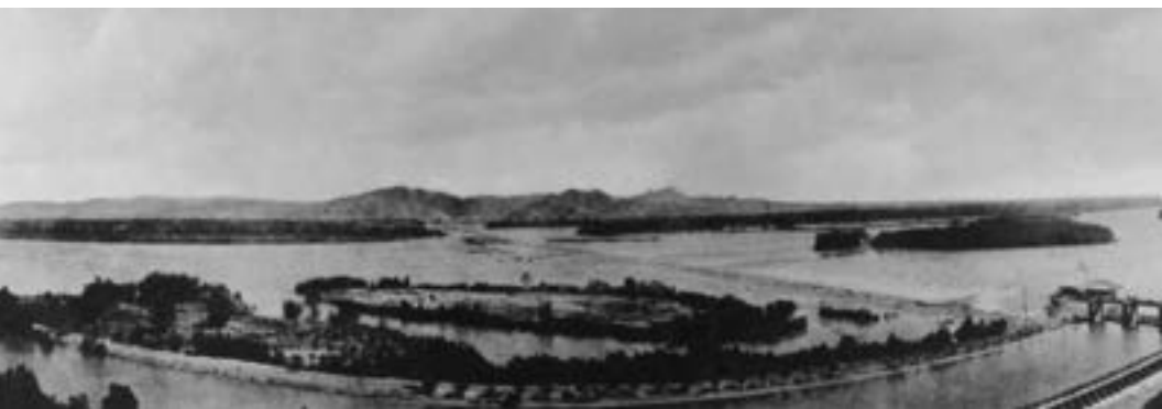
Yuma Projects Office Historical Photo 7-6 National Archives Photo (115-JAJ-781 Yum Box 309) Laguna Dam; view of California sluiceway below the gates. March 24, 1909
