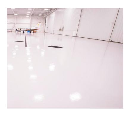
**RIOCOAT ECP** is a high solids epoxy coating that can be used on multiple surfaces. This resilient high-gloss surface is easy to clean and provides protection against wear and abrasions.
