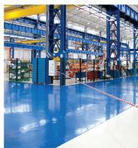
RIOCOAT UHW is a high solids moisture cured urethane coating. It can be applied clear or pigmented with no filler leaving a high gloss smooth finish, glass beads can be added to provide nonslip, better abrasion resistance with high gloss or aluminum oxide can be added to provide the highest abrasion resistance. The addition of more aluminum oxide will provide a satin finish while adding less will give a gloss finish.
