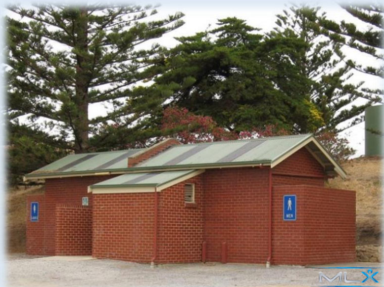
Picture: Toilet facities at rapid bay
